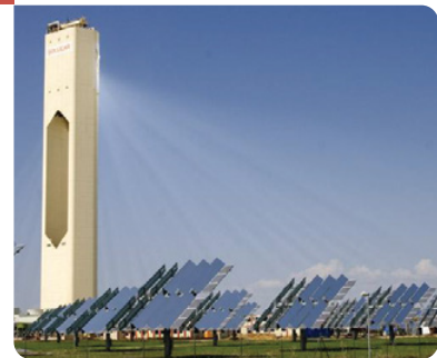
Power Tower Systems
